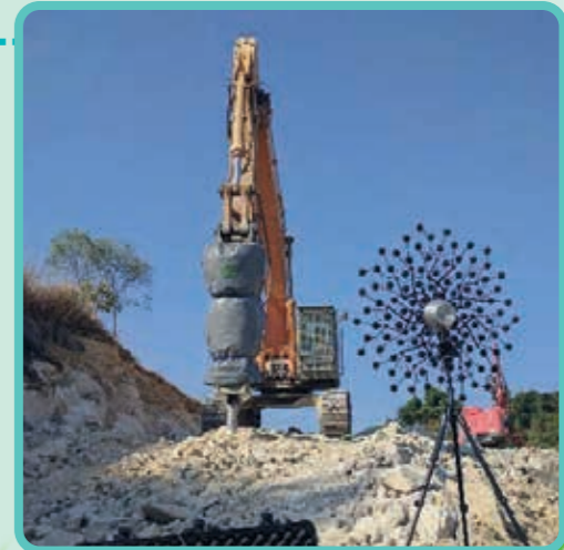
以隔音物料包裹打石機的機械式撞擊部份以減低噪音 Wrapping up the mechanical breaking parts of the breaker by acoustic materials to minimize noise nuisance
