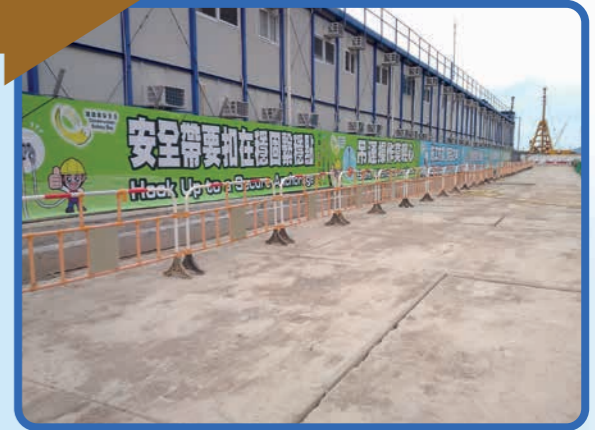
鋪設混凝土預製板以減少塵埃 Provision of pre-cast concrete units to minimize dusty problem
