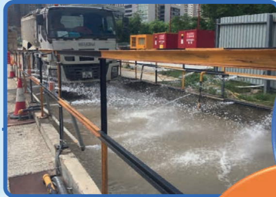
安裝自動清洗車輪系統 Provision of automatic wheel washing facilities
