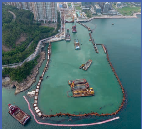
將軍澳灣填海工程進行中 Reclamation works at Tseung Kwan O Bay in progress
