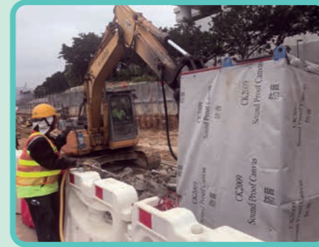
以隔音物料包裹打石機的機械式撞擊部份以減低噪音 Wrapping up the mechanical breaking parts of the breaker by acoustic materials to minimize noise nuisance
