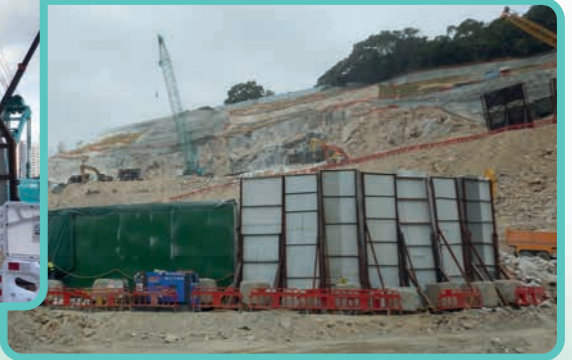
豎立臨時隔音屏障 Installation of temporary noise barriers
